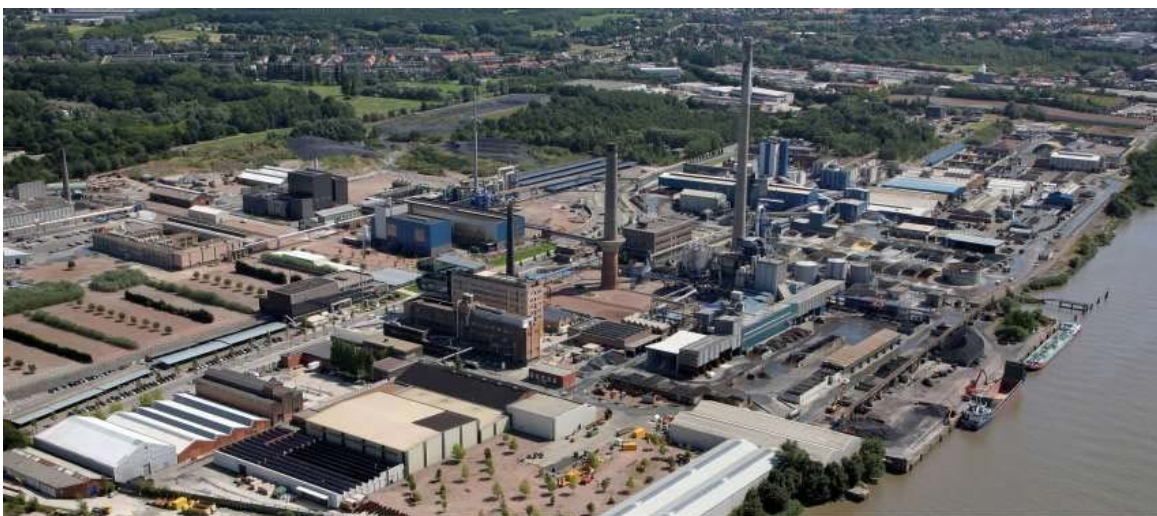
Figure 37 Umicore's integrated smelter in Hoboken, Antwerp. With a secondary material input of 350,000 t/year, it is the largest recycling plant of its kind in the world [Hagelüken, Treffer 2011]
